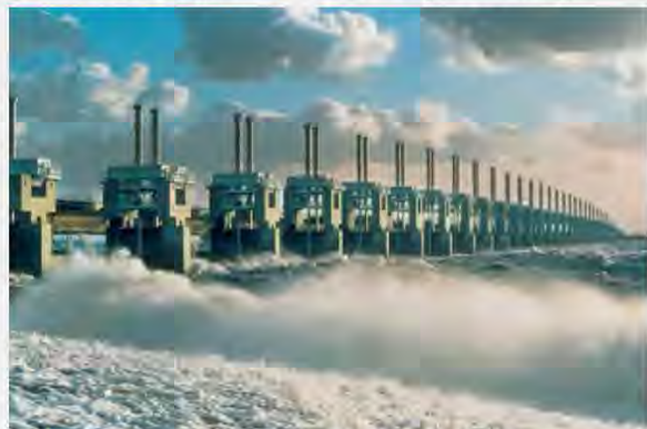
Photo 14: Maeslant storm barrier
